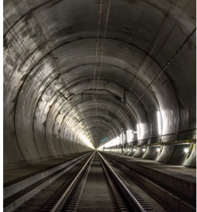
Semi-trailers with a 4-metre corner height can be transported through the Gotthard base tunnel.
