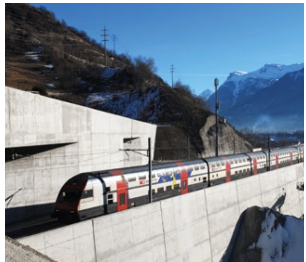
The Lötschberg base tunnel shortens journey times between northern and southern Europe.
