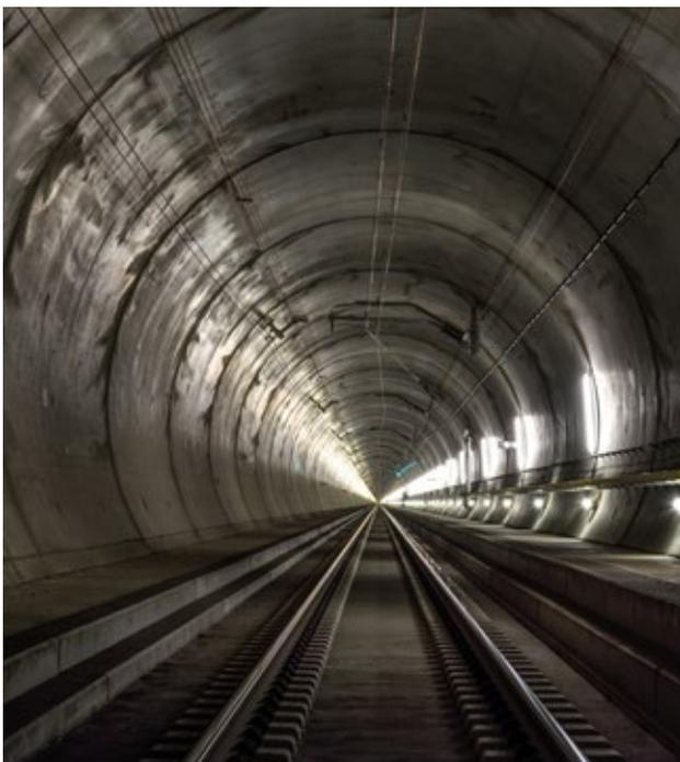
Semi-trailers with a 4-metre corner height can be transported through the Gotthard base tunnel.
